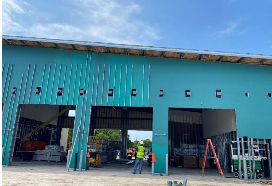
Current Building Front
