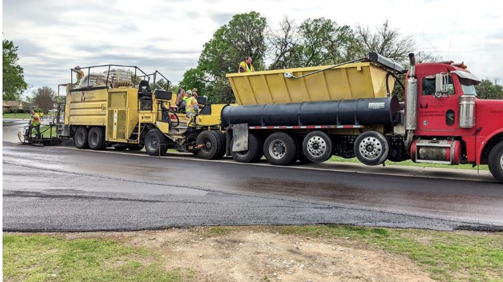
Viking Construction micro-surfacing Lodema Rd.
