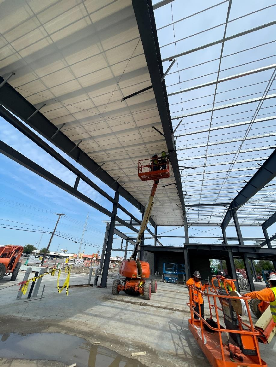
Fire Station 271 Roof Installation
