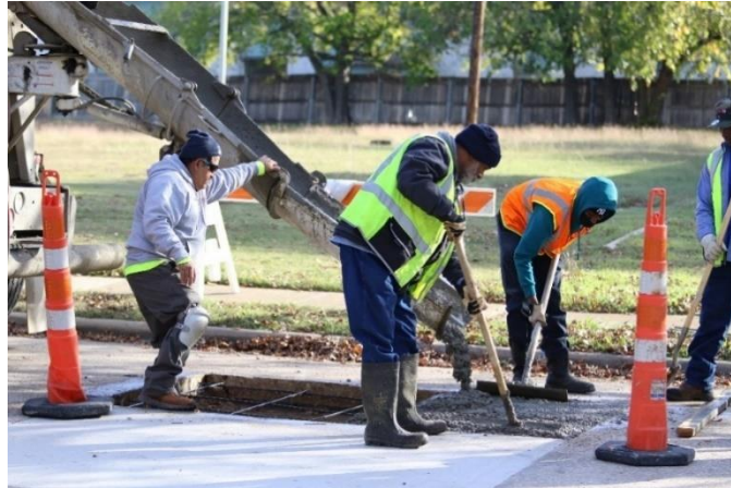
Utility repair on Power Dr.
