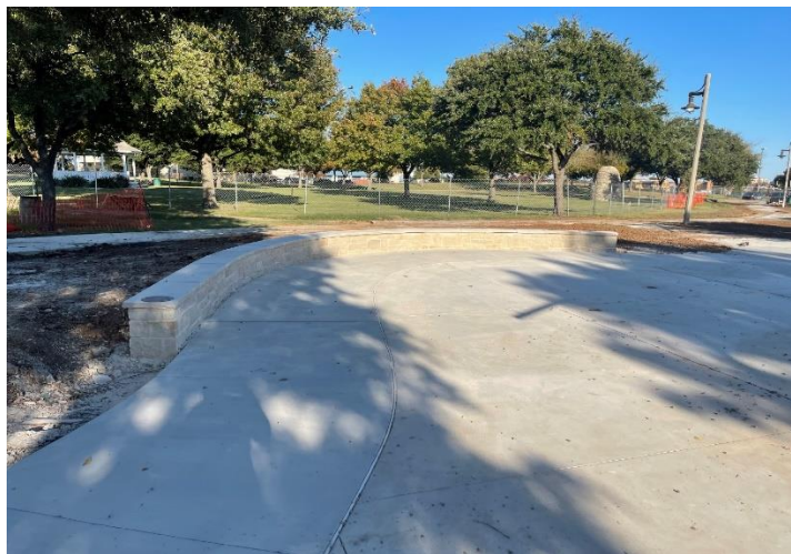
Splashpad pump house at Armstrong Park
