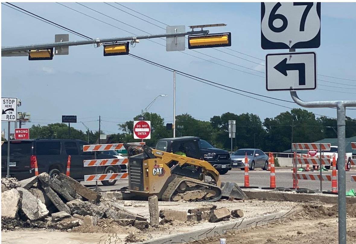
Debris Removal and Grading at U.S. Hwy. 67
