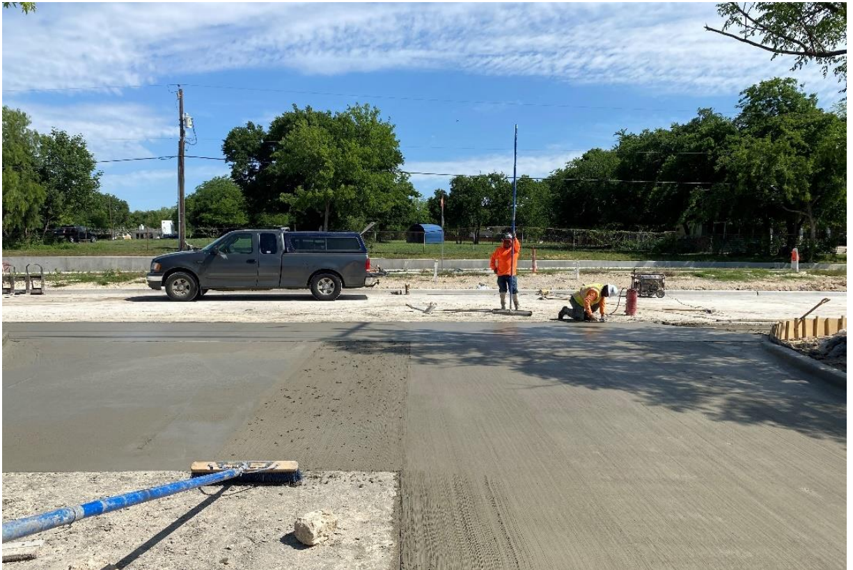
Sunrise Approach Concrete Placement
