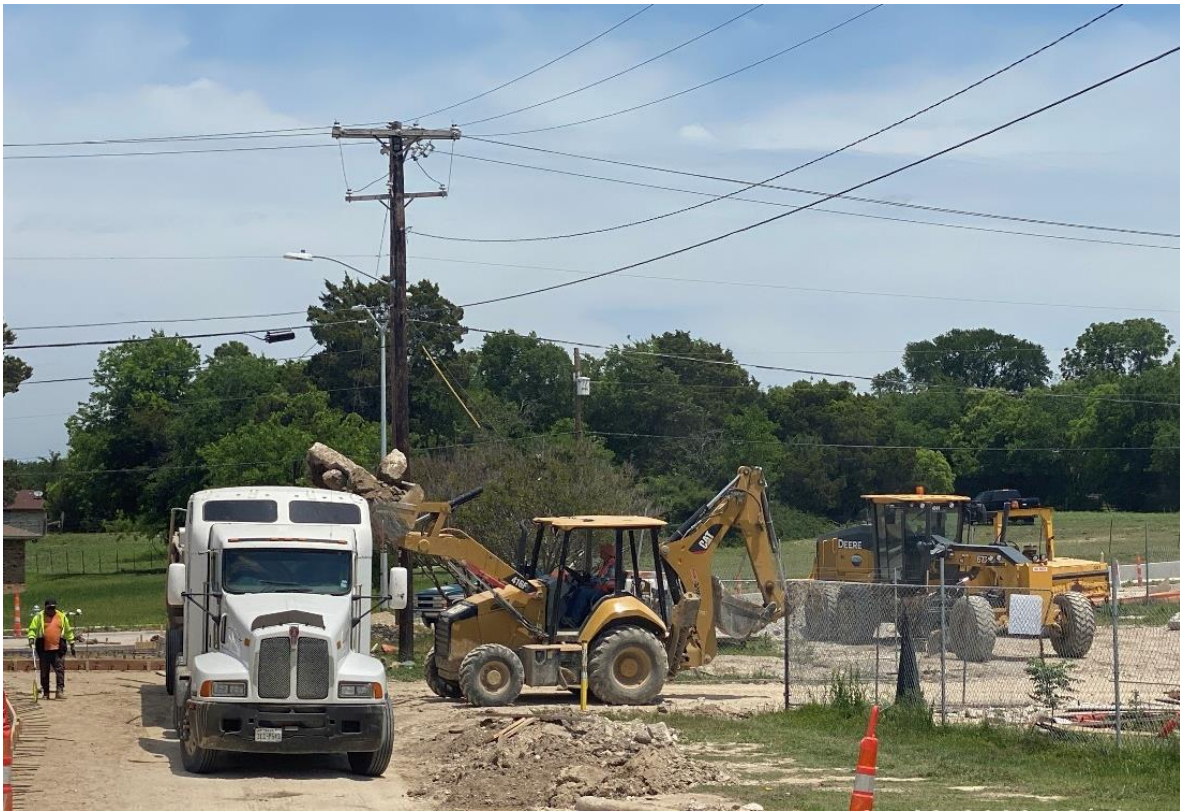
Concrete and Debris Removal from Bob Lee Drop Yard
