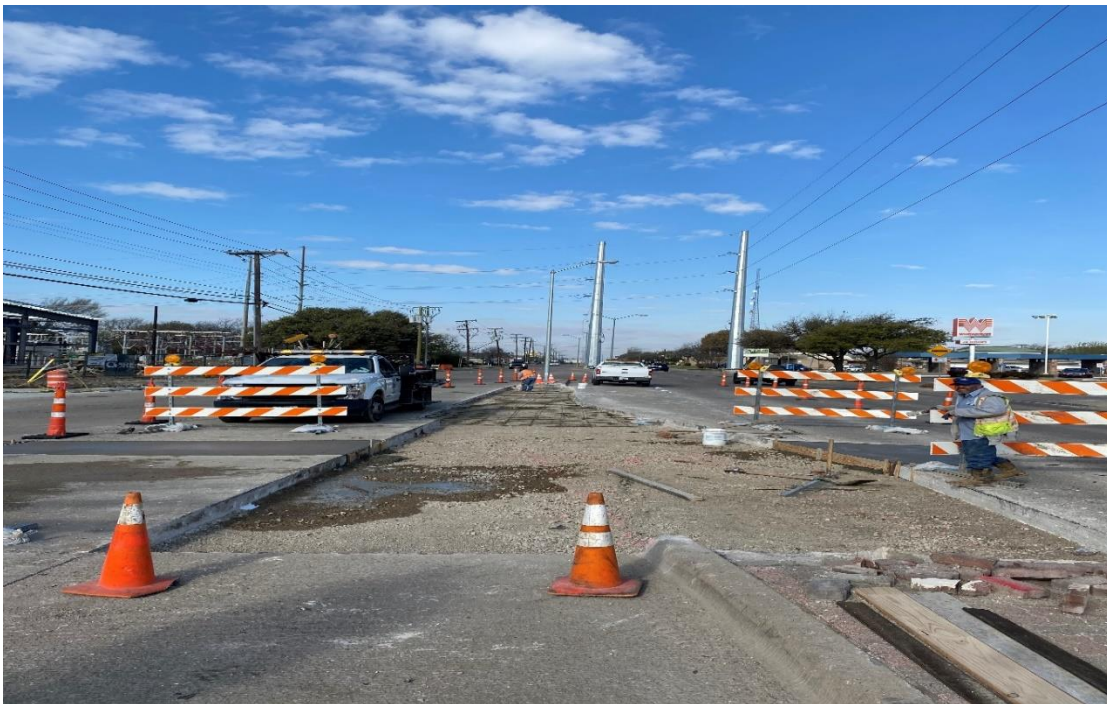
Removing Pavement and Median on Camp Wisdom Road
