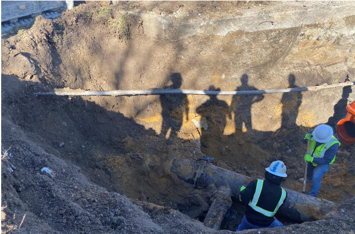
Danieldale Rd. - Abandoning the old water line at Water Line 4
